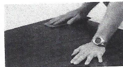
SAND TO REMOVE GLAZE AND IMPROVE ADHESION
