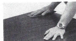
SAND TO REMOVE GLAZE AND IMPROVE ADHESION
